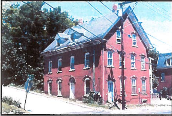
Historic building and apartment house in need of restoration; note brick deterioration and eave / roof repair needs.
